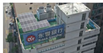
► The rooftop solar PV system at Bank SinoPac Beigao building.
